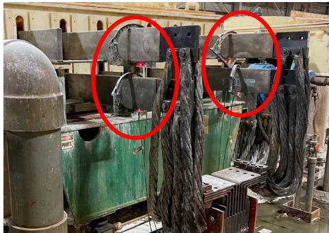
CPCO – Current Probe, Clamp-on Probe based on same technology and design with larger aperture, in use at an electrochemical plant.
